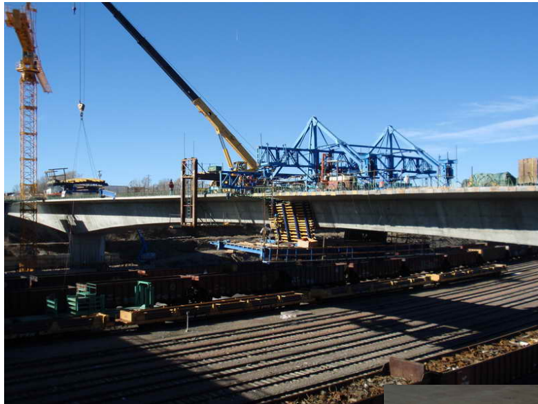
Figure 3 – Cantilever 4 WB Segmental Construction – December 1, 2009:
