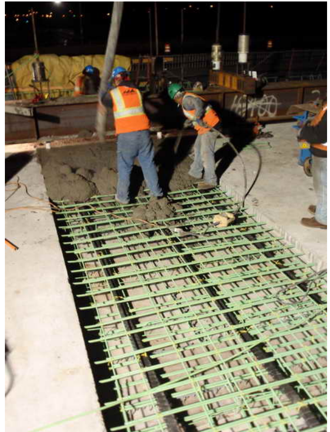
Figure 8 – Span 4 WB Closure Segment Construction – December 16, 2009: Concrete is placed and finished for the top slab of the closure segment at Span 4 WB
