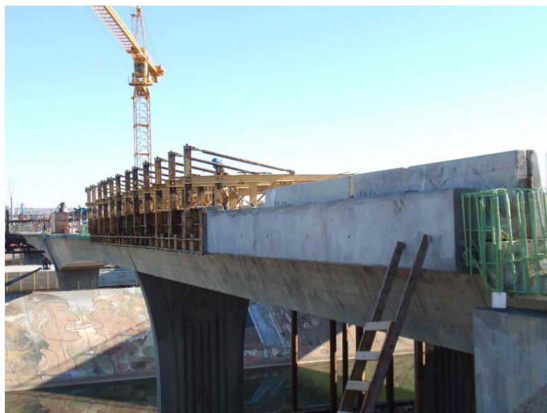
Figure 2 – Cantilever 4 WB Segmental Construction – November 30, 2009:
