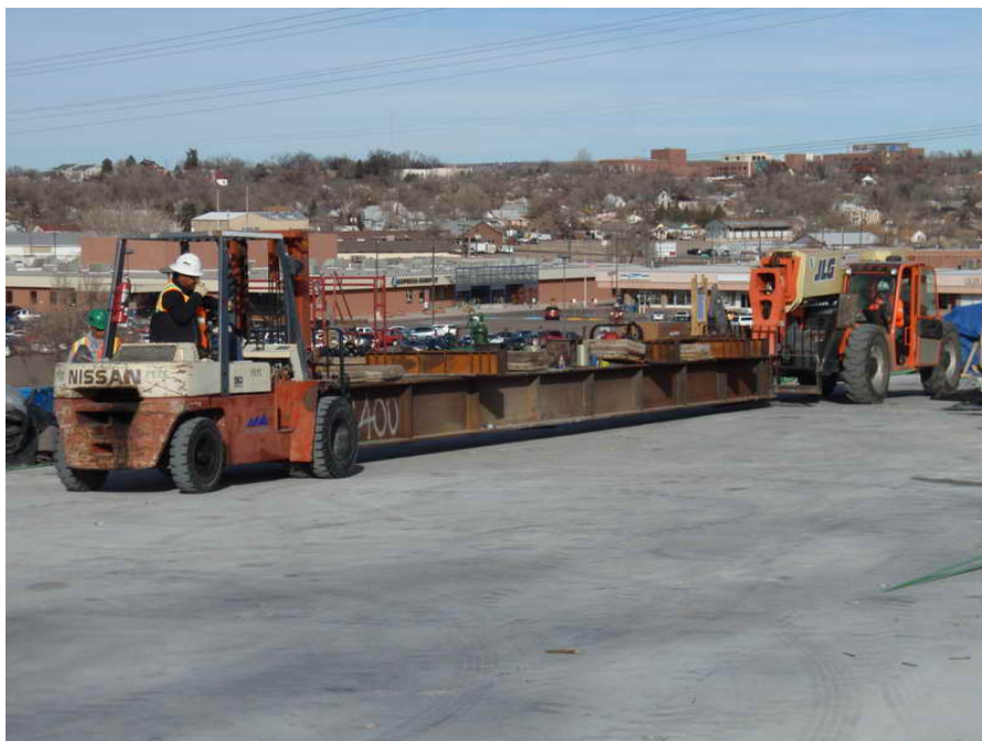
Figure 15 – Span 3 WB Closure Segment Construction – December 21, 2009: The strongbacks are transported across the deck from Span 4 WB to Span 3 WB closure joint using two forklifts. Once the strongback was near the Span 3 closure segment, the 50-ton crane picked the downstation end as the forklift held the upstation end to span the gap across the closure. These beams cannot be engaged until all stressing is complete in Span 4 WB, which is anticipated tomorrow.
