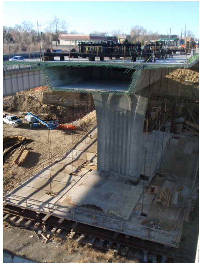
Figure 10 – Span 1 EB CIP Superstructure Construction – December 17, 2009: The second portion of the falsework removal process is complete with the lowering of the remaining three falsework spans. The pedestrian trail was closed for the falsework removal and is scheduled to be reopened upon cleanup.
