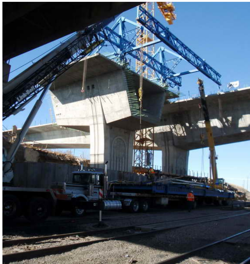
Figure 7 – Cantilever 3 EB Segmental Construction – December 15, 2009: The form traveler crew prepares the lower deck drive for a tandem pick. Once the lower deck drive was near the bottom slab of the pier table, the chain hoists were engaged and were used to set the lower drive to the proper elevation.
