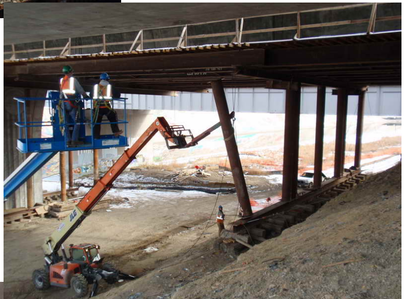
Figure 4 – Span 1 EB CIP Superstructure Construction – December 11, 2009:
