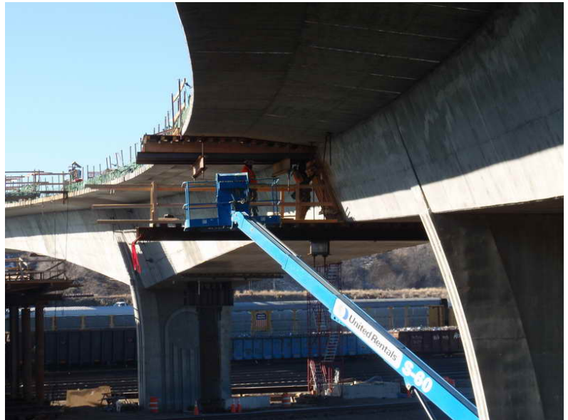
Figure 6 – Span 4 WB Closure Segment Construction – December 15, 2009: Workers install the web form ties at Span 4 WB closure joint. The stability prop can be seen in the background.
