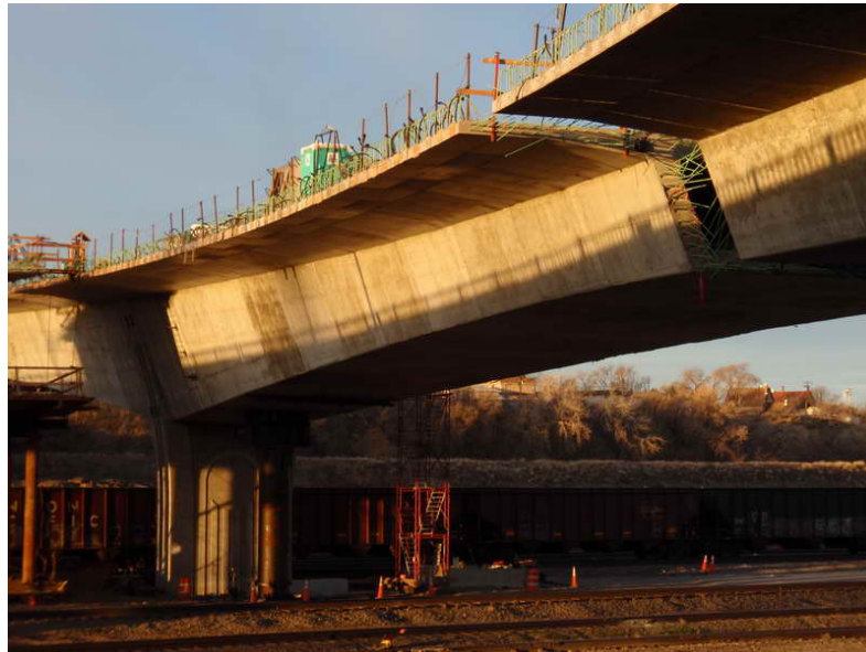
Figure 1 – Cantilever 4 WB Segmental Construction – November 25, 2009:
