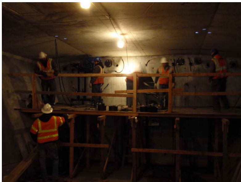
Figure 11 – Span 4 WB Closure Segment Construction – December 17, 2009: The PT crew stresses the 19-strand longitudinal draped tendons for Span 4 WB.
