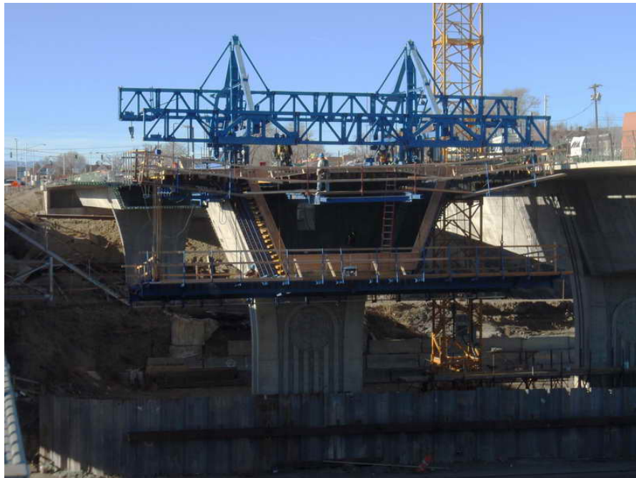
Figure 14 – Span 4 WB Closure Segment Construction – December 21, 2009: Forming for Segment E3-1E is nearly complete with the bulkhead installed. Reinforcing installation began today.
